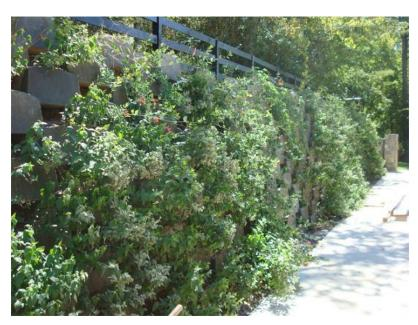
A GreenWay installation can range from 70 degrees inclination (20 degrees of batter) to 50 degrees inclination (40 degrees of batter). Thus, design flexibility offers application as segmented retaining wall or slope stabilization, always with the intention of full vegetated cover.
